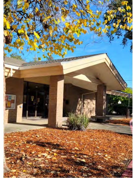
Cloverdale Regional Library front entrance
