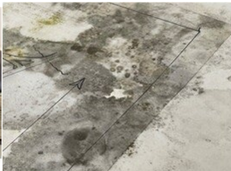
Inactive mold is dry and powdery
